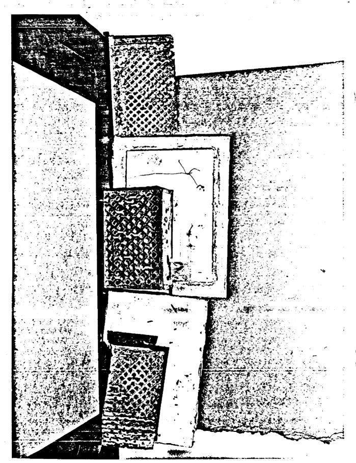
Rear view of three replicas of ventilator grills used by Subjects to replace original grills in their three cells. Note wire hooks by which grill and surrounding surface could be pulled into place after Subject's exit into the utility area.
