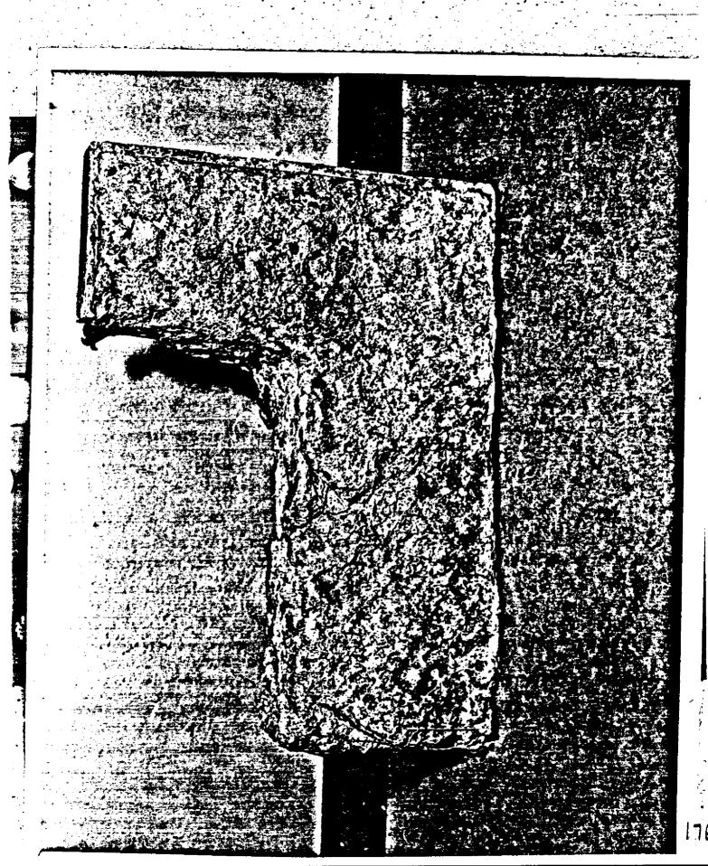
Concrete replica: this is the reproduced utility wall surface made to replace the concrete removed in order avoid detection by a guard check along the utility corridor. This concrete was applied to hard board. (Photo by SA [6/14/62]
