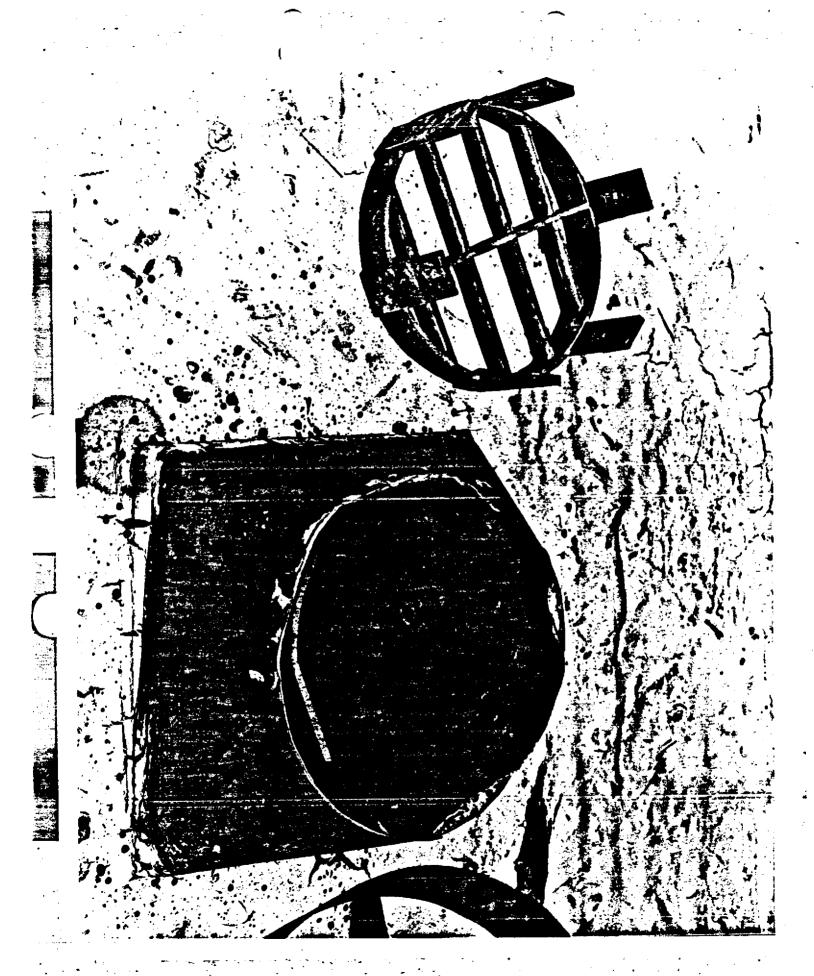
1-4 Photo taken by photographer standing on pipe vent shown in 1-1 looking into the galvanized vent leading into space over Cell Block B. Photo taken in an eastern direction and shows one of the two re-enforcing rods which obstructed this hole and was bent to permit egress.
