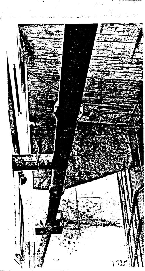
2-7 Photograph taken by leaning over the edge of the building showing the bake overn stack extending from above the roof line to the clean out on the concrete slab at ground level. The edge of the building is at left center and the distance from this to ground level is approximately forty-five feet. The wire screen topped with barbed wire seen at lower right is approximately twelve feet high.
